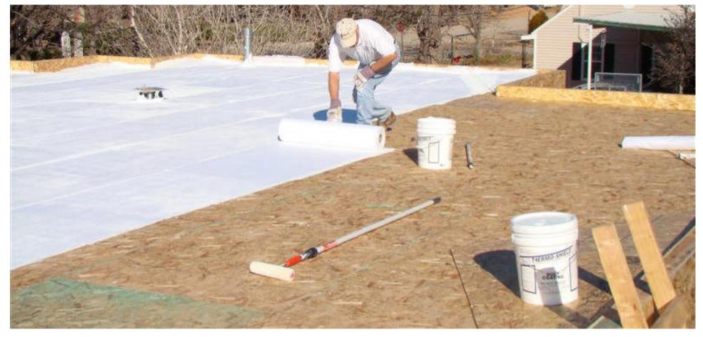
The Thermo-shield Rep advised me to simply lift the loose areas and apply more Thermo-shield under the fabric and brush the fabric down. Worked great. Got the second coat on and another bigger storm soaked the area but not one drop got in my house
