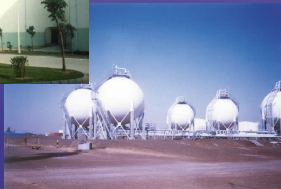
Natural Gas Tanks, Tianjin, China
