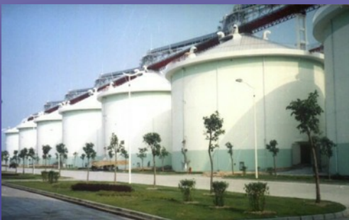
National Grain Barn, Guangzhou China
